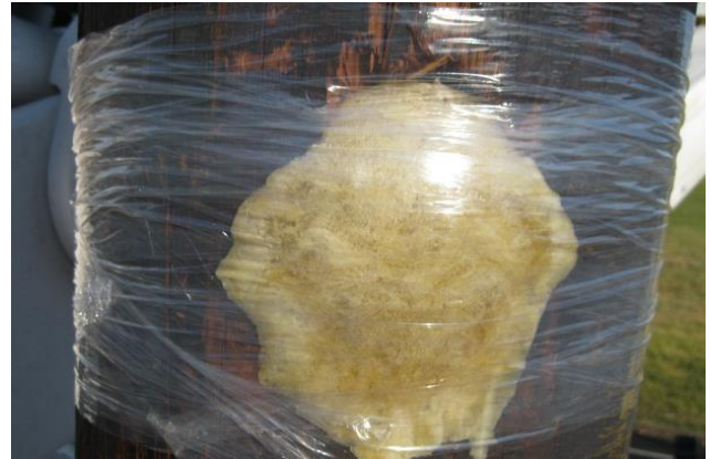
Woodpecker damage repaired with UPR™ Pole Repair
